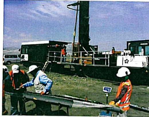
Sonic drill rig at Guadalupito.
