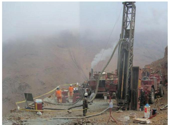
“All of the original drilling intersected oxidised rocks, so our aim with the diamond drilling is to get behind and underneath those early holes and try and get into the sulphide part of the system.”
