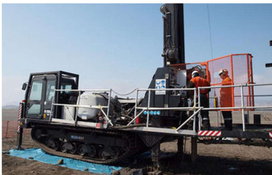
Site works at Latin Resources' Guadalupito project.
