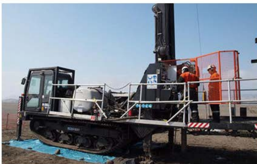
Site works at Latin Resources' Guadalupito project.
